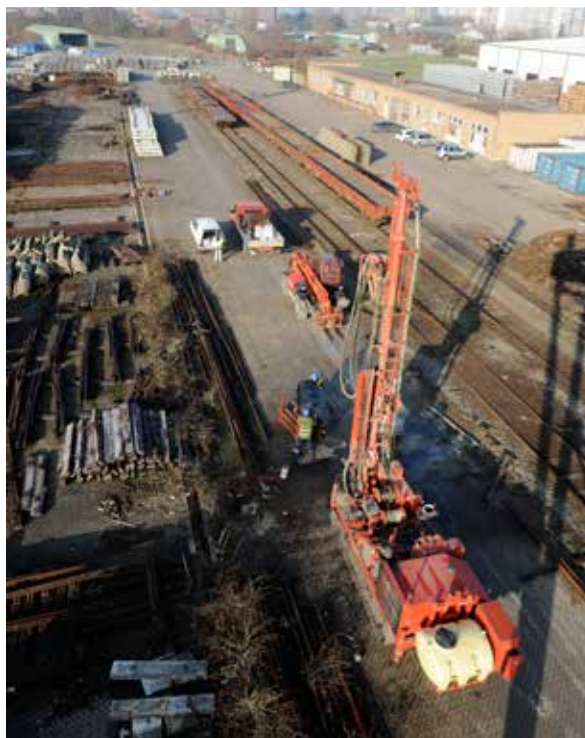
Soil sampling on the "Cour aux marchandises SNCB" site, Bressoux, for the Liege tramway construction project
